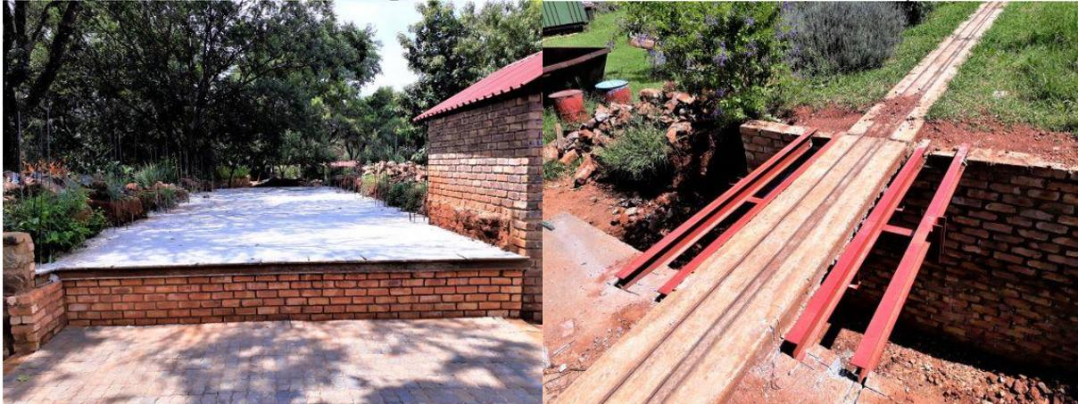
air supported by the generous use of reinforcement in the concrete. A steel structure has been fabricated from steel in our stock to form a new bridge to support and carry the track over the culvert. We are hoping the project will be completed for March Track Day.
