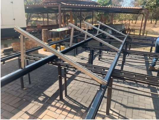
Frames for the additional solar panels done.
