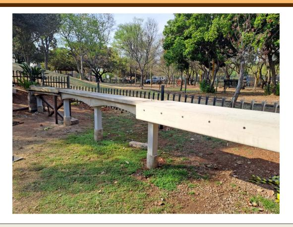
The bridges from the 45mm station platform to the tunnel are being replaced with solid in-situ concrete castings. The project is aimed to simulate the Gautrain bridges at the Jean Avenue crossing, and to make them strong enough to withstand the might of the Hennops in flood! We are also installing 'permanent' aluminium track from the tunnel to the northern side up to the small bridge.
